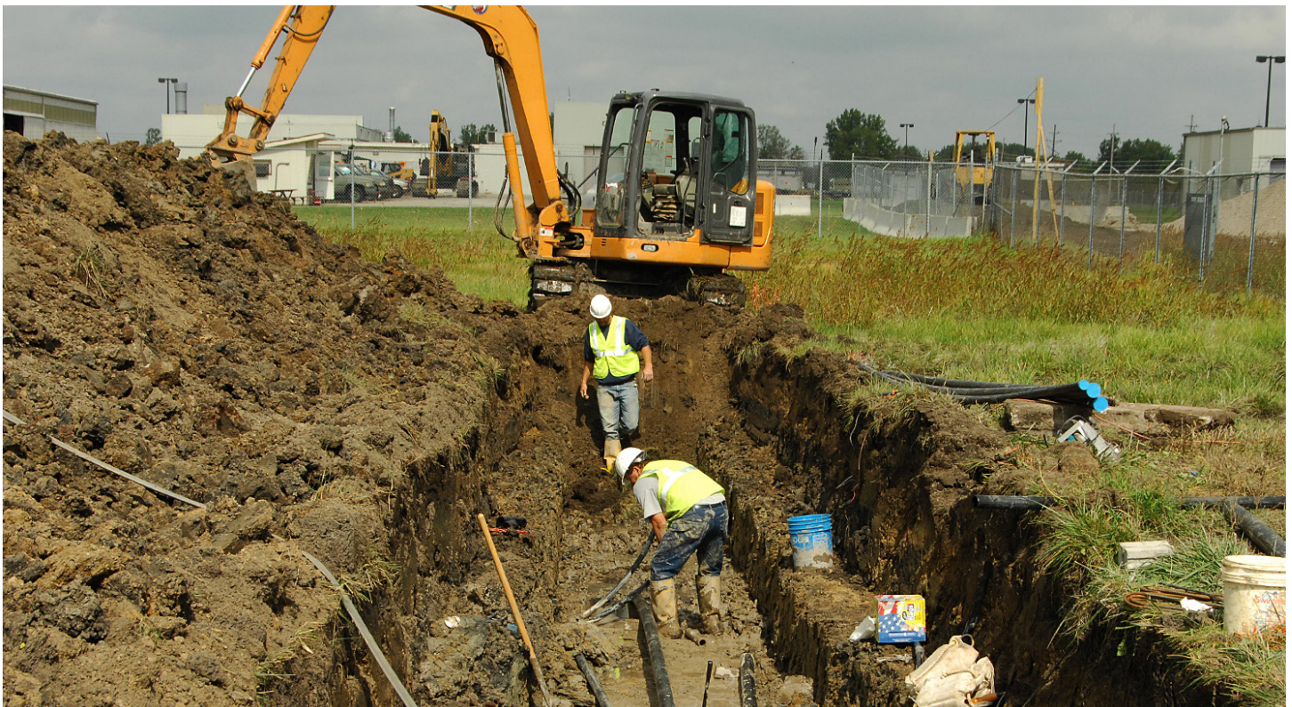
Workers prepare to splice a “T” pipe while installing a geothermal system at Selfridge Air National Guard Base, Michigan, September 29, 2011. (Department of Air Force photo by John Swanson)
