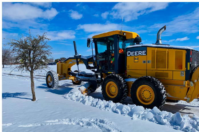
A member of the 17th Civil Engineering Squadron enhances the safety of travel routes by clearing snow at Goodfellow Air Force Base, Texas, February 15, 2021. The 17th CES adapted and overcame the challenges of record-breaking snowfall with no proper removal equipment in order to continue the mission. (Courtesy photo)
