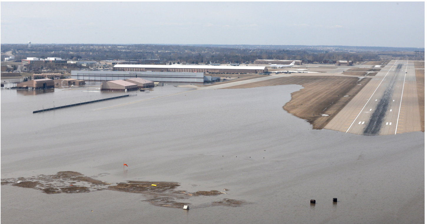
March 2019 flooding at Offutt Air Force Base, Nebraska, limited runway use, even after floodwaters receded, due to inspection requirements. The new STRATCOM headquarters building, completed earlier in 2019, was built on higher ground, with barriers to reduce flood risk, and thus was not affected by the flooding. (Department of Air Force photo by Tech Sgt Rachelle Blake)
